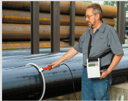
Porosity detection on pipelines
