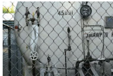
Difficult inspection sites
